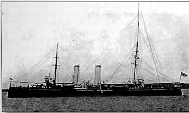
H.M.S. Thetis showing her extended main mast carrying the wire aerial
